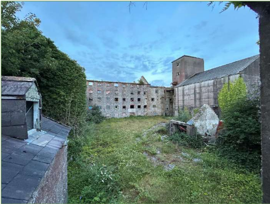
A1. View from Easthill House, looking towards Mill Buildings.
