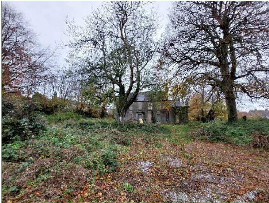
A3. View of Rosehill House.
