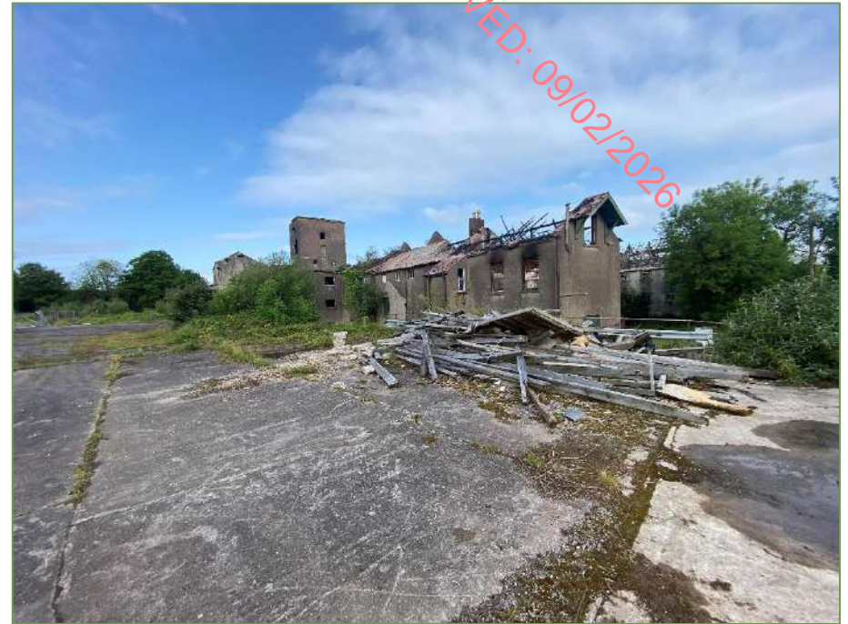
A2. View of Mill Buildings from east.
